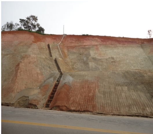
Drainage systems. Protection of a slope in the side of Tamoios highway
